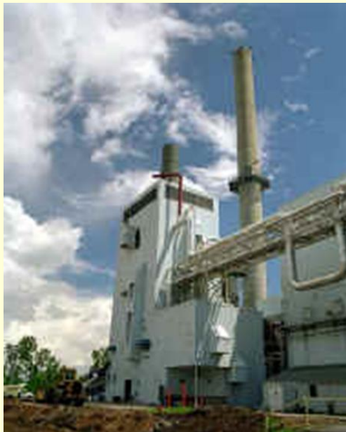
5 MWt Woodchip Bubbling Fluidized Bed Gasifier (Vermont)
